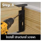
**WARNING:** All connector hole locations must be filled with proper screws for safe and correct installation. **DECK JOISTS SHOULD NOT BE STEPPED ON OR LOADED** before all screws are installed into the connector.
