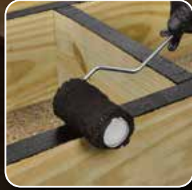
Deck Frame Coating 2025
