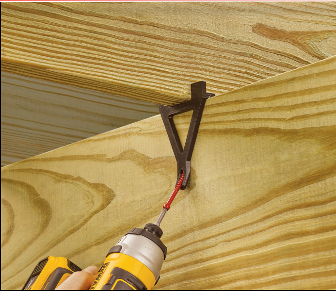
Deck Joist to Carrying Beam
