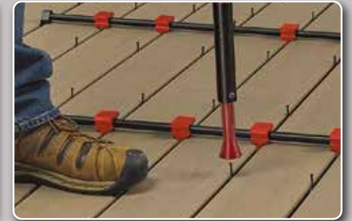
3) Install clips with ZipStick
