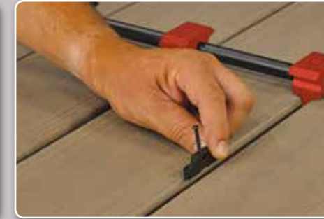
2) Place ZipClips in board gaps
